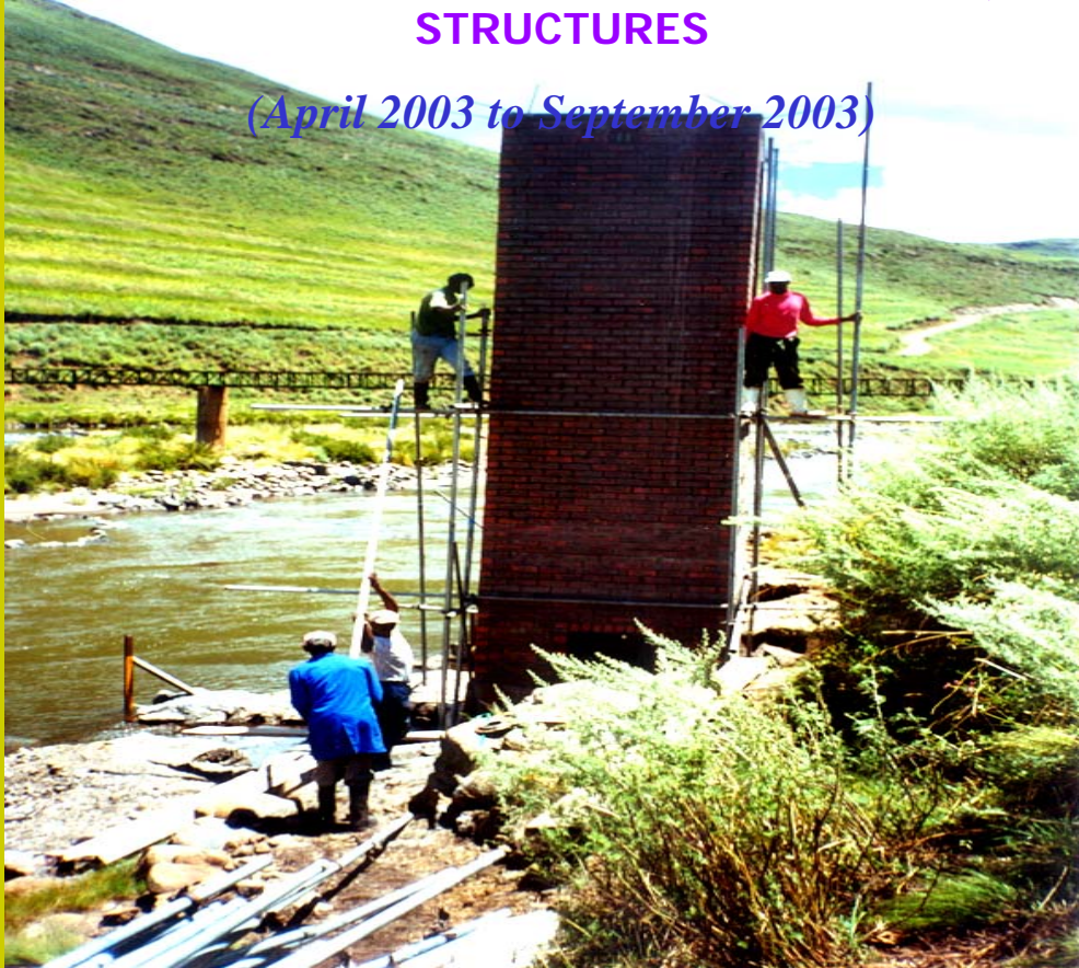
TOWER ON MALIBAMATSO RIVER @ KAO
